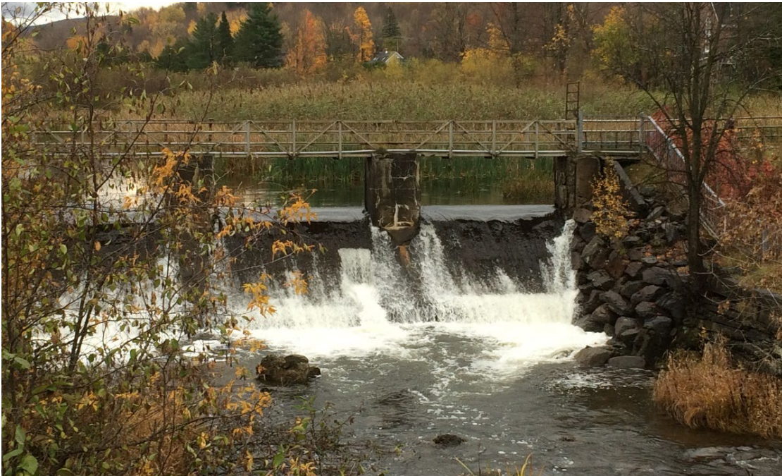
Figure 18 – Le barrage Blackwood
